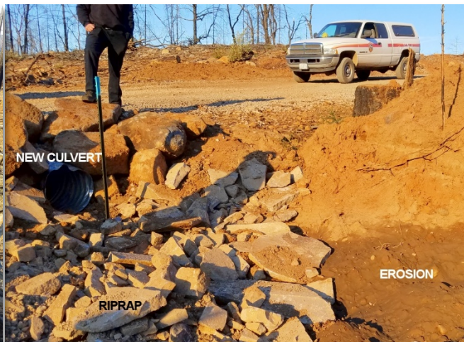
Quarried rocks are used as riprap to trap sediment at the entry of a new culvert. Photo: G. Stahl
