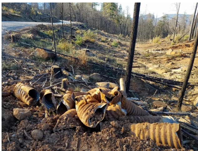
Old, rusted culverts have been replaced to manage flooding and runoff during the winter. Photo: G. Stahl
